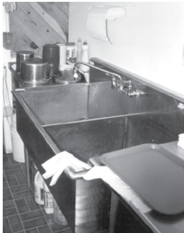
A ware-washing sink should have two or three compartments that are large enough to accommodate the immersion of equipment and utensils.
