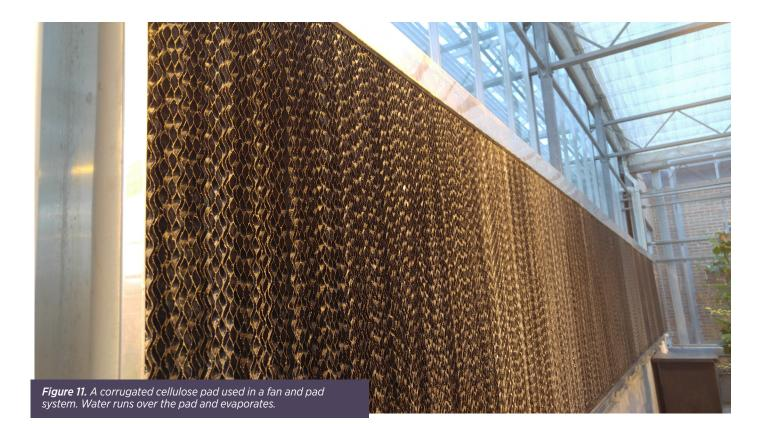
pulling the cooler air through the greenhouse. The exhaust fans pull air in through the inlet vents located on the opposite side of the pad and the air pulled across the pads passes through the length of the greenhouse. This cooled air rises in temperature as it passes through the greenhouse, so the pad end of the house is generally cooler than the fan end. This heat gain can be calculated and the distance between fan and pad are carefully managed according to climate requirements.
