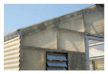
*Figure 7. Fiberglass reinforced plastic greenhouse material that has degraded in a way that greatly reduces light transmission.*
