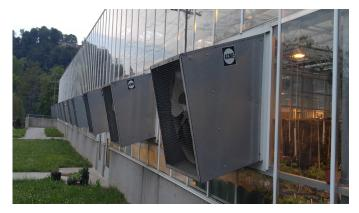
**Figure 10.** Evaporative cooling is accomplished as an exhaust fan pulls air out of the greenhouse and pulls air through a pad on the other side of the greenhouse. These fans are available in many sizes to fit a range of greenhouse structures.
